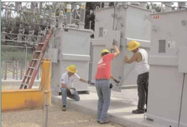
**At Left** | Corn Belt Power electricians install a transformer at the Fern Substation. This new substation, located near the intersection of Highways 20 and 14, serves the new Grundy County Heritage Center, a member of Grundy County REC.
