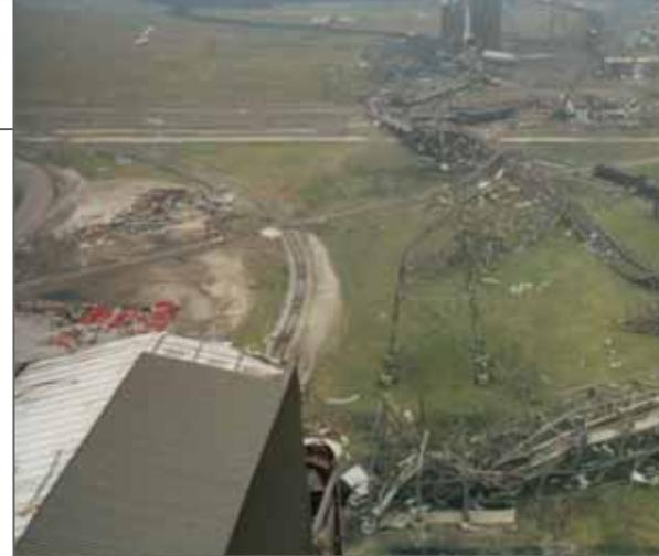
**Above** | A tornado that hit the Neal 4 power plant 20 years ago on July 28, 1986, destroyed the plant's coal handling equipment and blew away 75 percent of the turbine building roof. The facility was brought back on line 300 days later.
