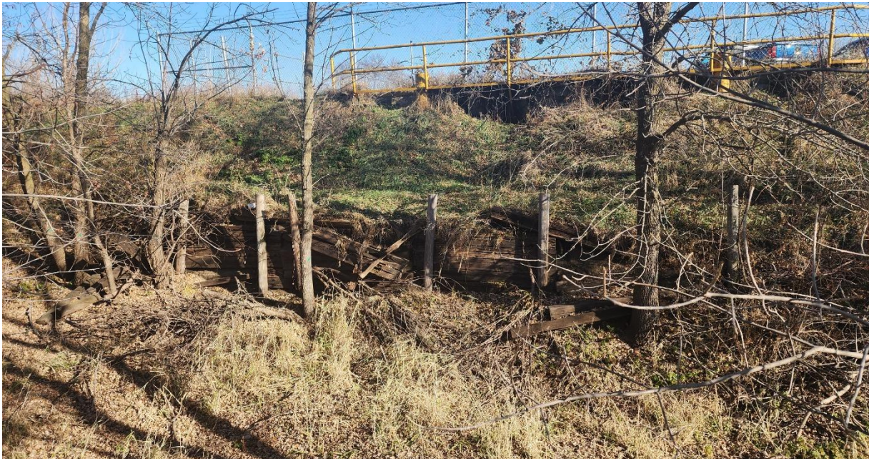
Photo 4 Support structure on north side of ash pond, viewed across the ash pond. Looking north.
