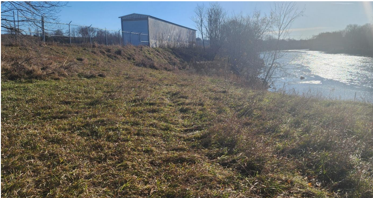
Photo 2 Grade outside north end of ash pond. Looking east.
