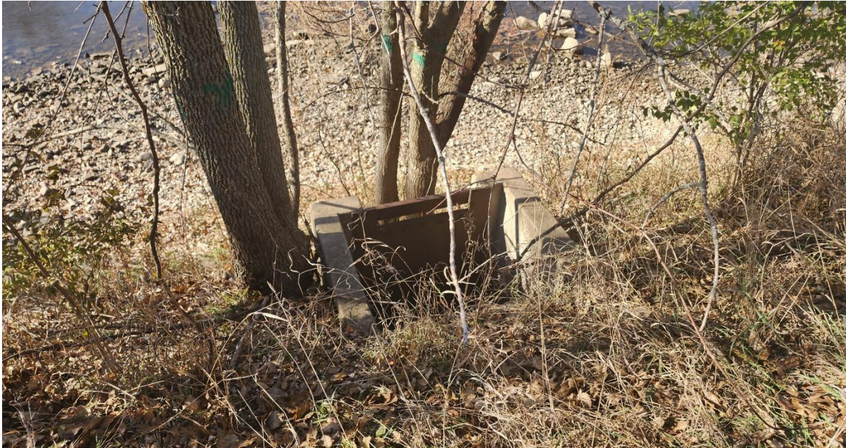
Photo 3 Former outfall structure along river bank, south of ash pond, near north end of ash pond.
