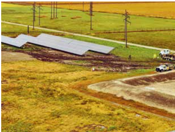
Top: Corn Belt Power's new solar array at Wisdom Station features 600 total panels, totaling 150 kilowatts of renewable generation.
