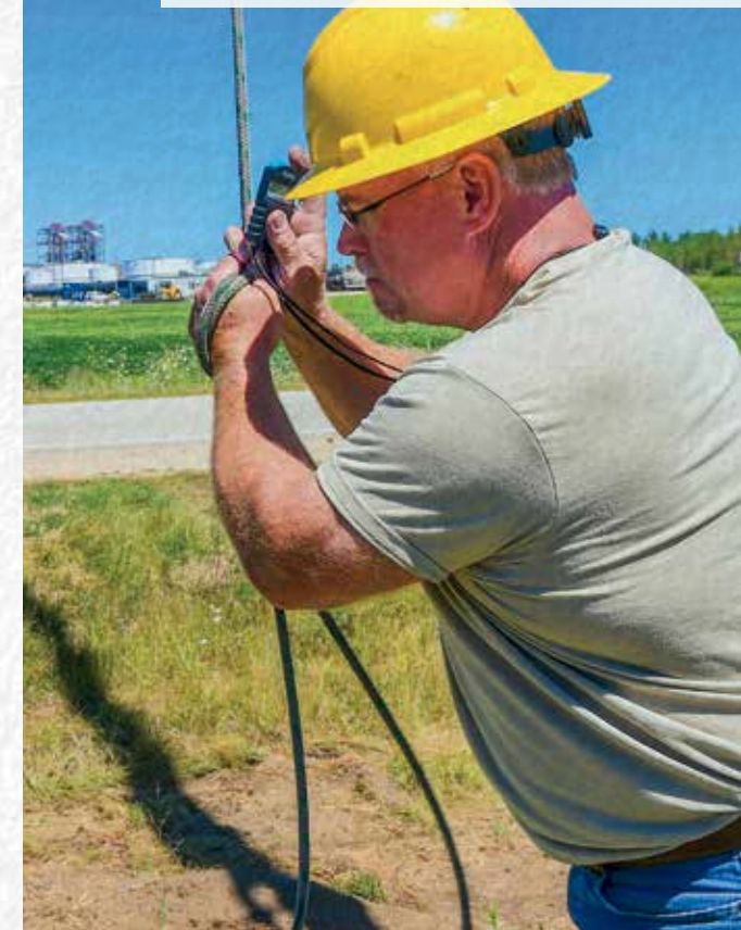
Corie Erickson, assistant right-of-way and land supervisor, determines line tension along the Bauman Tap in the Butler Logistics Park.
