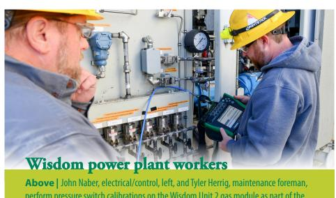
perform pressure switch calibrations on the Wisdom Unit 2 gas module as part of the preventative maintenance program.
